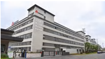
High-tech Zone Factory
